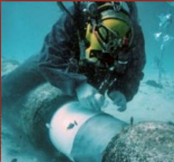
PIPELINE CONCRETE REMOVAL FOR NDT TEST
