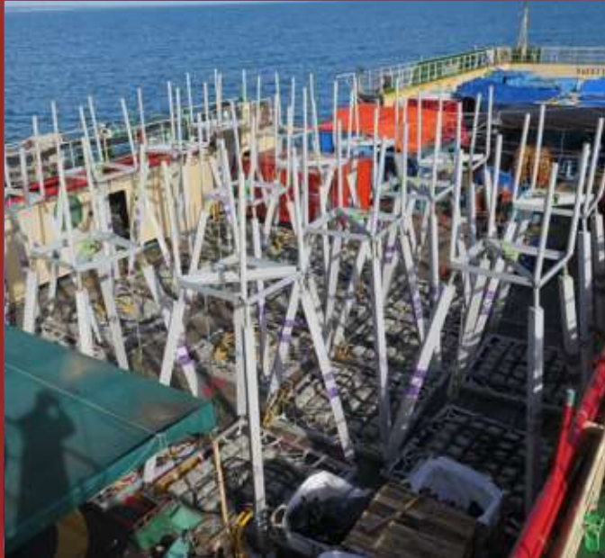
CP ANODE POD'S ON DECK
