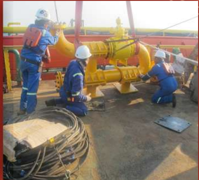
INSTALLATION OF SPOOL PIECE AT PLEM
