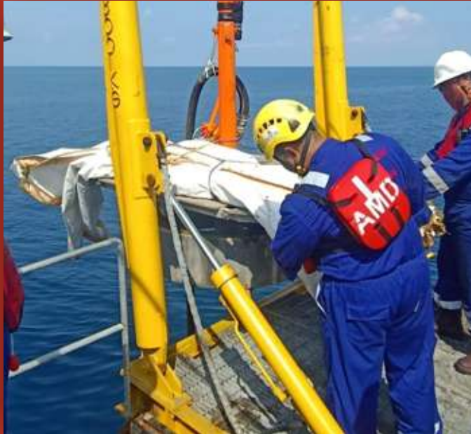
DEPLOYING GROUT BAG TURNTABLE
