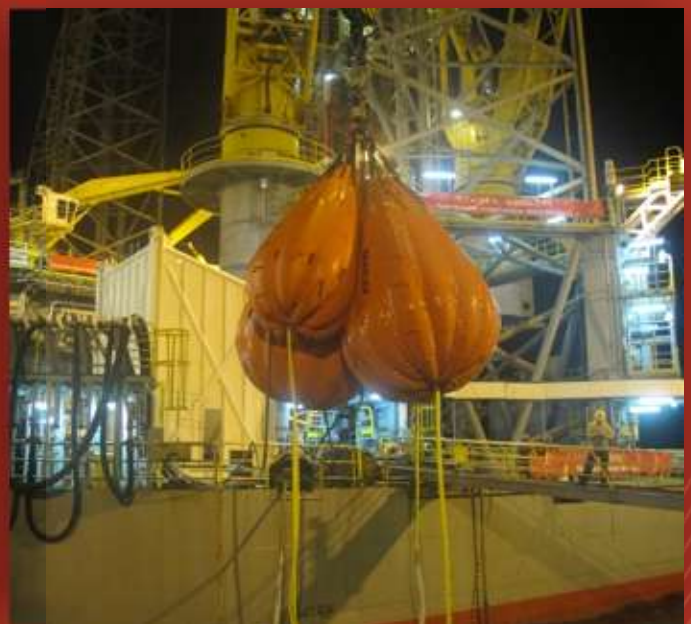
CRANE LOAD TEST JACK UP RIG HYSY 937
