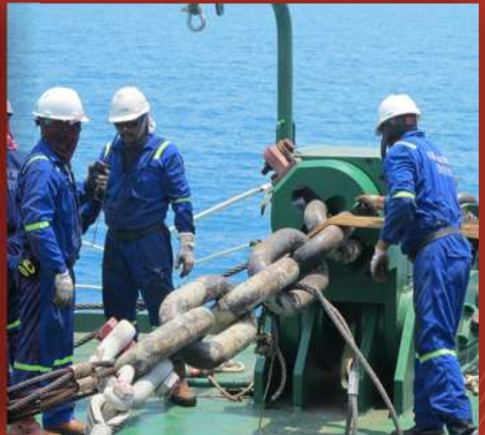
INSTALL CHAIN TO CHAIN STOPPER
