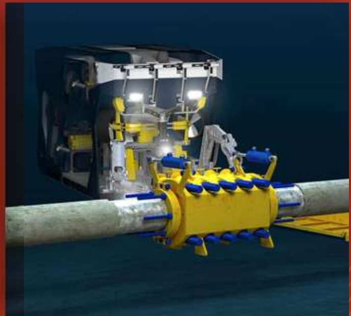
PLIDCO CLAMP INSTALLATION BY ROV WORK CLASS
